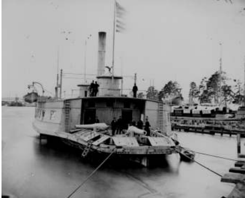
No known pictures exist of the USS Fort Henry . This is the USS Commodore Perry , the same type of fore-and-aft ferry boat.
